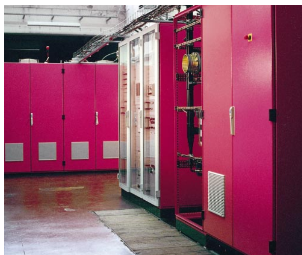
FIG 4 75 kW klystron amplifier system (500 MHz) for scientific applications
